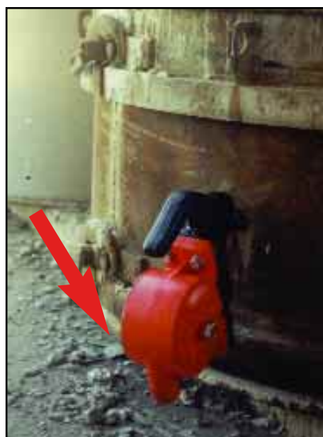
Silent pneumatic turbine model VS-510 on wedge bracket on well liner form.
