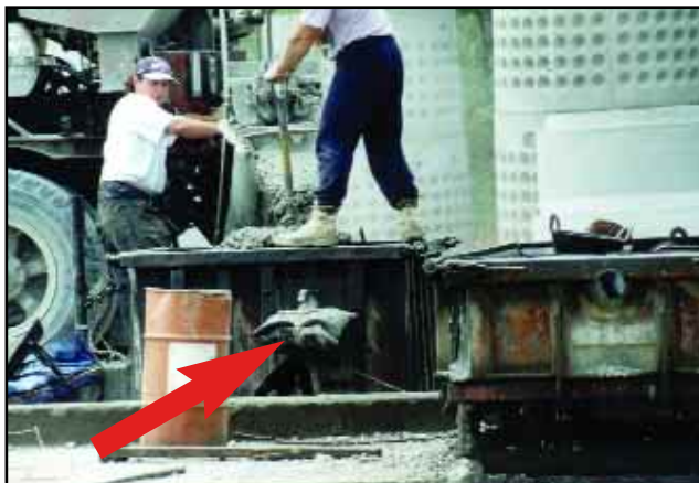
US-1600 with wedge on culvert form. (Notice a rubber sheet covers vibrator and protects it from concrete spill.)
