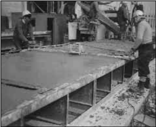
Model 2P-800 on 8' screed, made from a 6" channel iron with adjustable rods to minimize the bowing of the screed.
