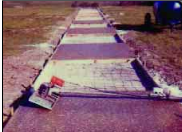
Finished sidewalk after it is washed.
